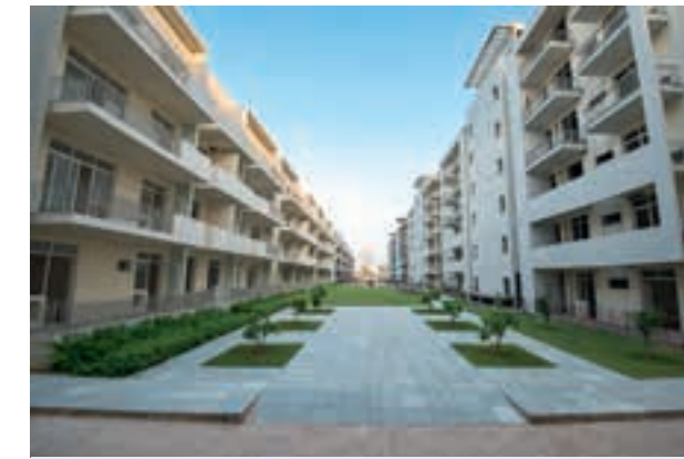
Over 200 families have already settled. 560 units are ready for possession out of 1150 apartments under construction
